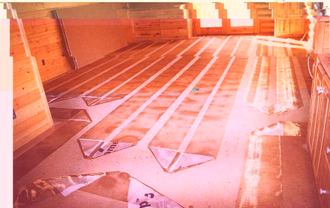
▲ Jensen Residence, Smith & Morehouse ▲ Screen on wood sub-floor - under wood floor and carpet
