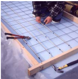
Floorizwarm Heating Element Layout
