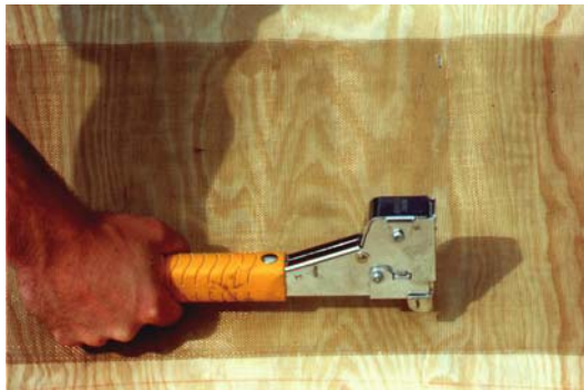
Illustration 2.45 Stapling Z Mesh.
