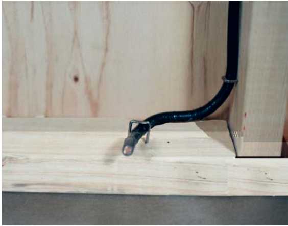
Illustration 2.38 Cold Lead rough-in for wall installation of Transition Plate.
