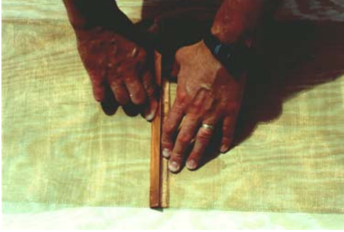
Illustration 2.50 Splicing of Z Mesh. Z Mesh being placed in fold of Splice Plate.
