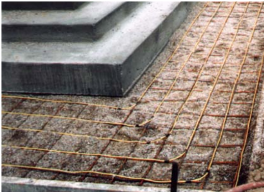
Illustration 2.2 Tuff Cable snow melting installation on stairs and landing. Tuff Cable is attached to welded wire fabric. Always jumper under joints of any kind—never run Tuff Cable through any kind of joint.
