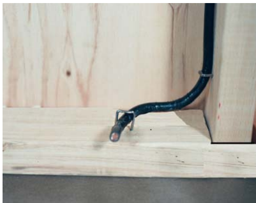
Illustration 1.8 Cold lead roughed-in for wall installation of Transition Plate (E217).
