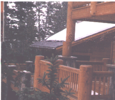
Roof de-icing with Z Mesh under asphalt shingles.
