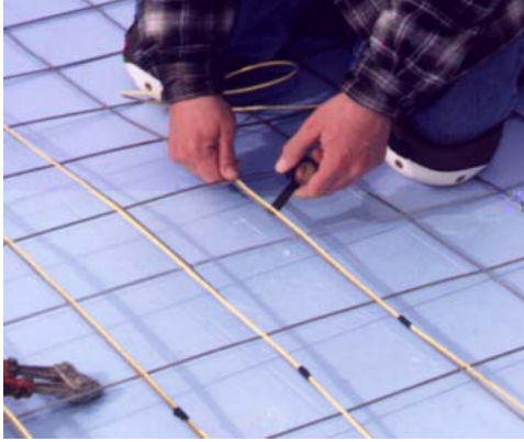
Illustration 2.4 Installation of Tuff Cable. Electrical tape or plastic wire ties must always be used to secure Tuff Cable to welded wire fabric.
