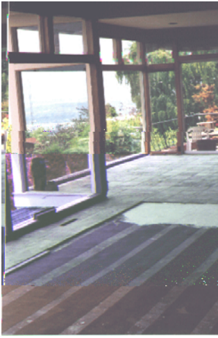
Z Mesh used in space heating of a sun room under tile.
