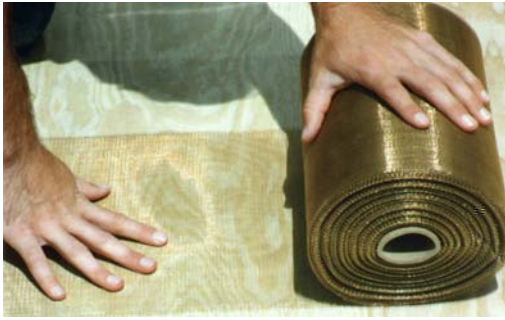
Illustration 2.43 Rolling out Z Mesh.
