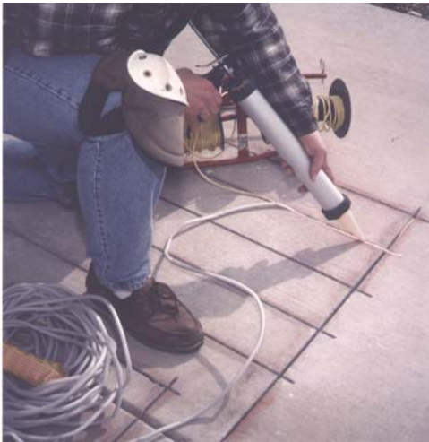
Illustration 2.21 Filling saw-cuts of retrofit installation.
