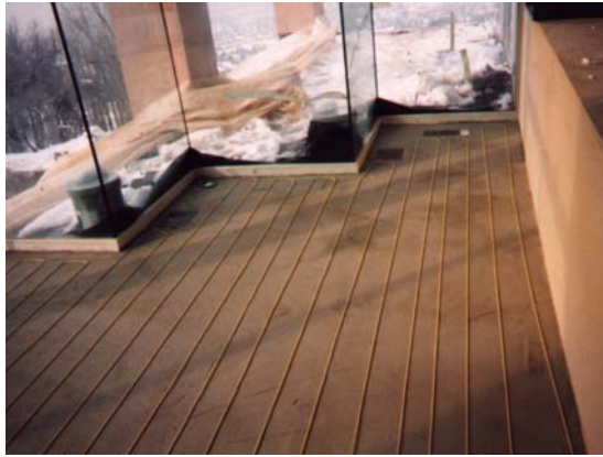
Illustration 2.1 Tuff Cable installed on top of mortar bed in space heating installation. Tuff Cable will be covered with thinset mortar prior to floor covering installation.
